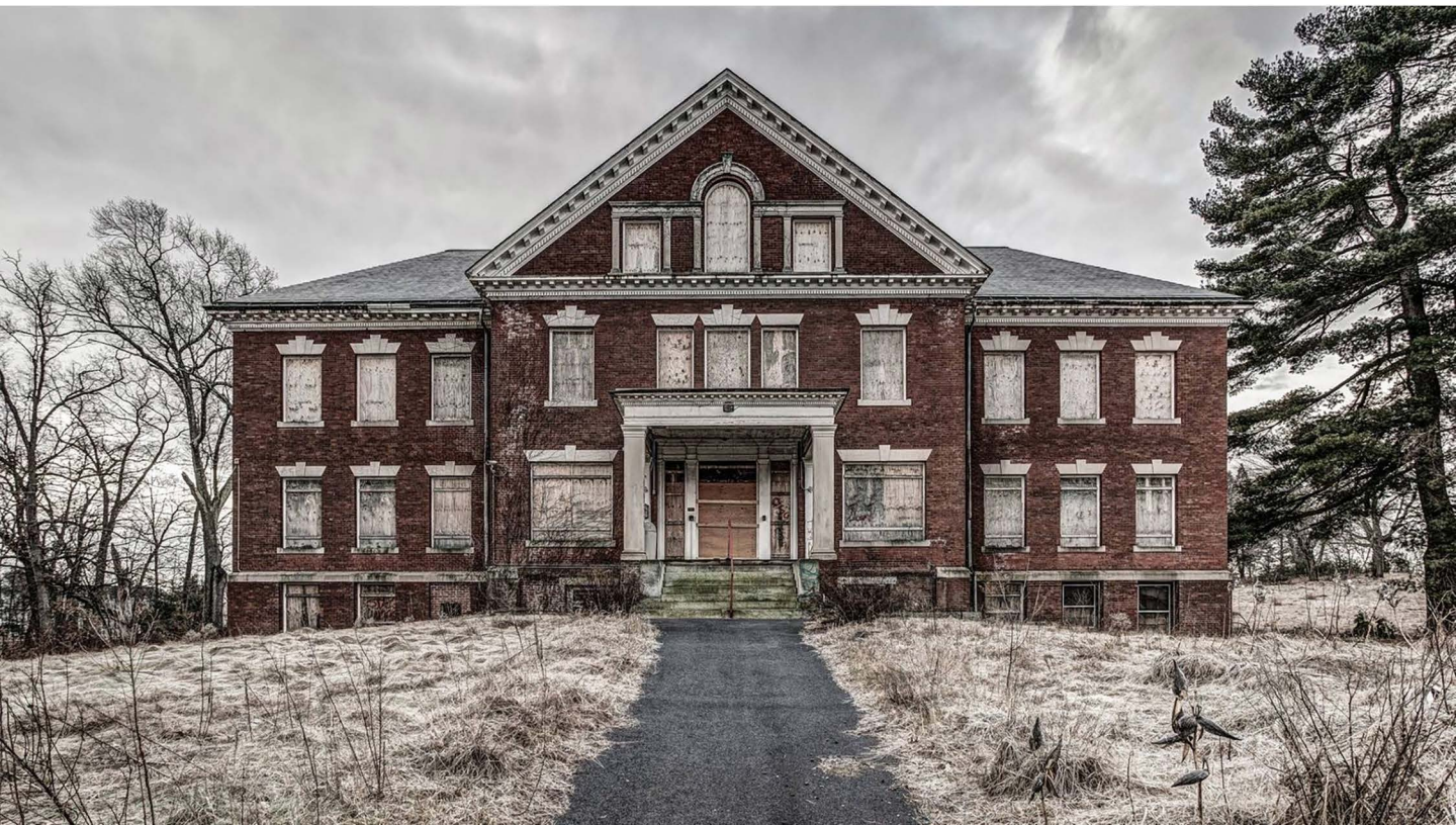
Bigelow Hall boarded up and abandoned, January 2019, posted by Mark Duffy
