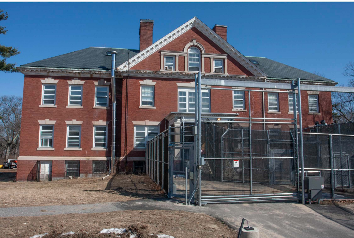
Bigelow Hall rear view, showing brand new fenced enclosure, March 14, 2009
