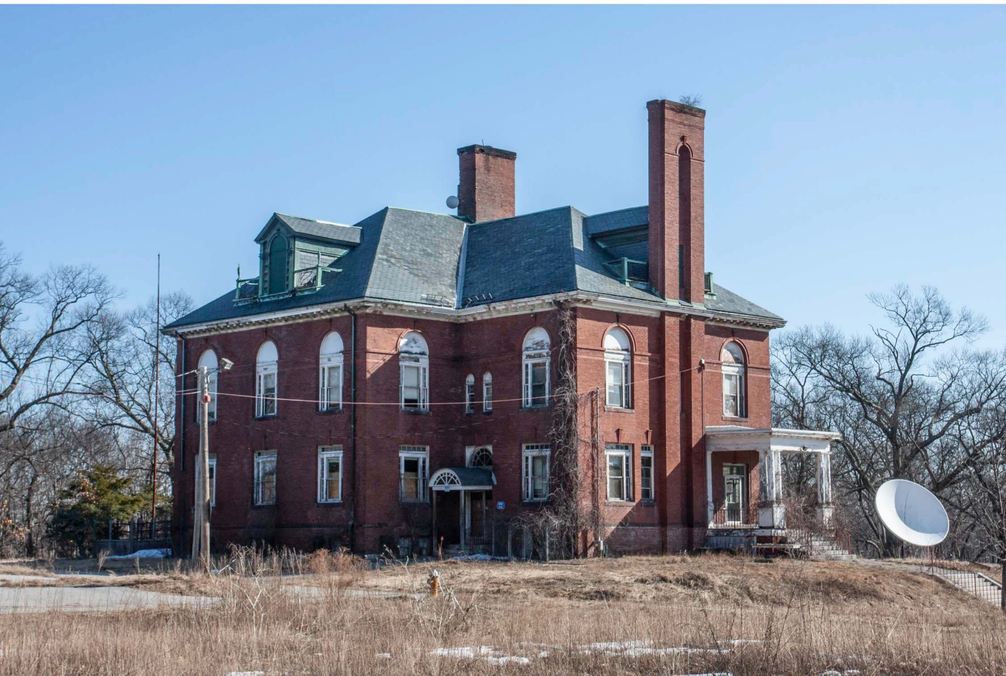
Front left view of Read Hall, grass on chimney and satellite dish, March 14, 2009
