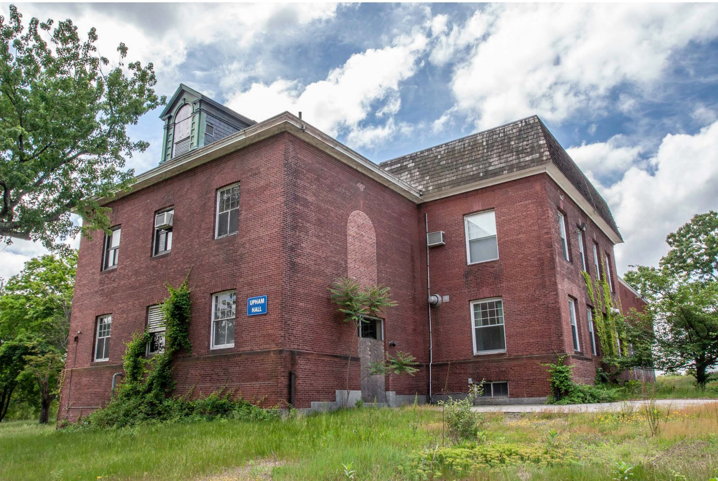
Upham Hall with new roofline, closed openings, and rear addition, June 10, 2007
