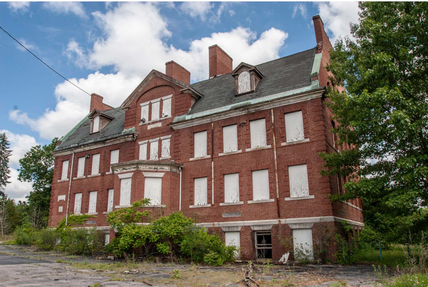
Abandoned Richardson Hall left rear, open window in basement, June 10, 2007
