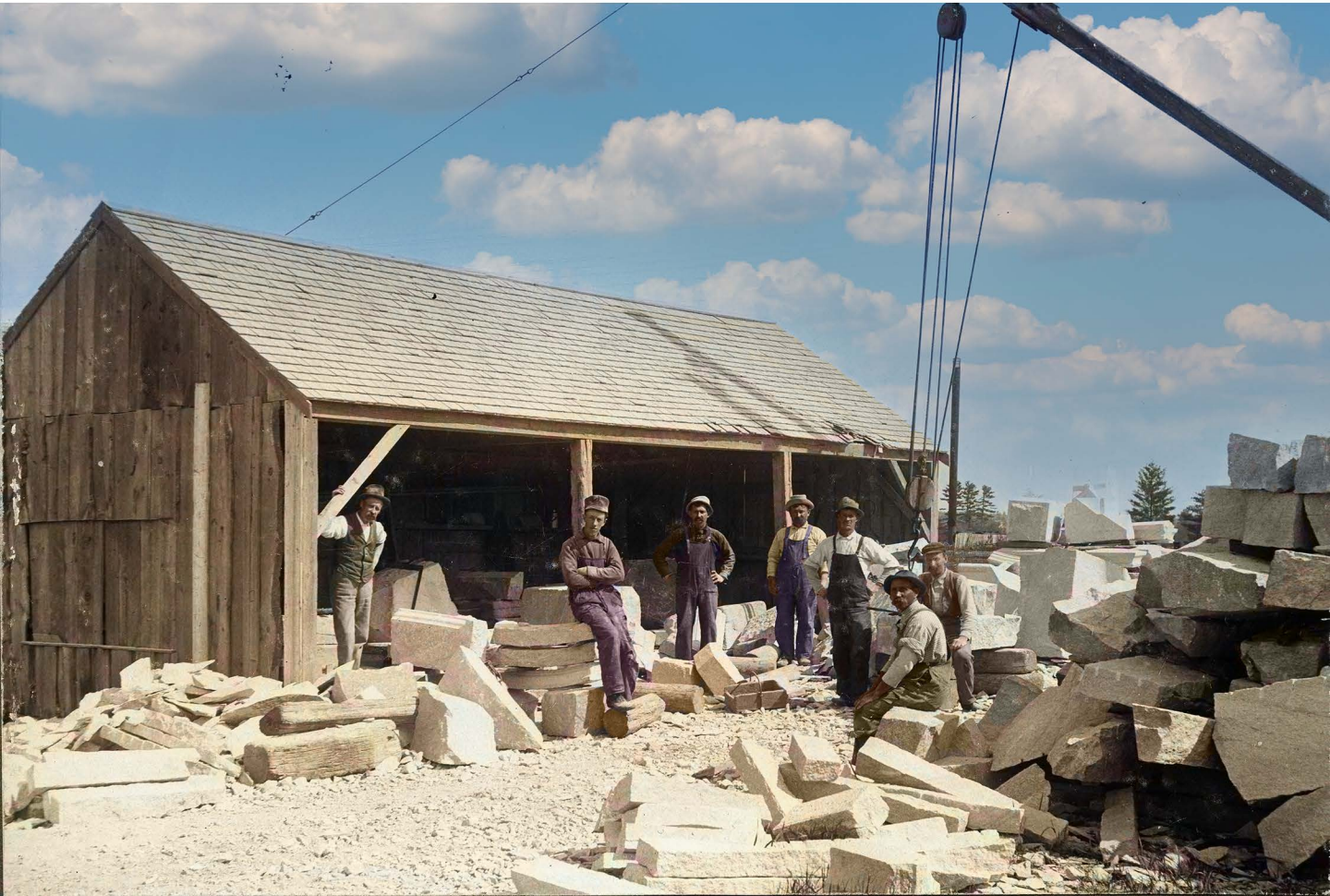
North Chelmsford's Marinel and Willsted Stone Works provided granite foundations for the Middlesex County Truant School. Courtesy of the Chelmsford Public Library
