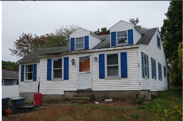
View looking southeast toward facade.
