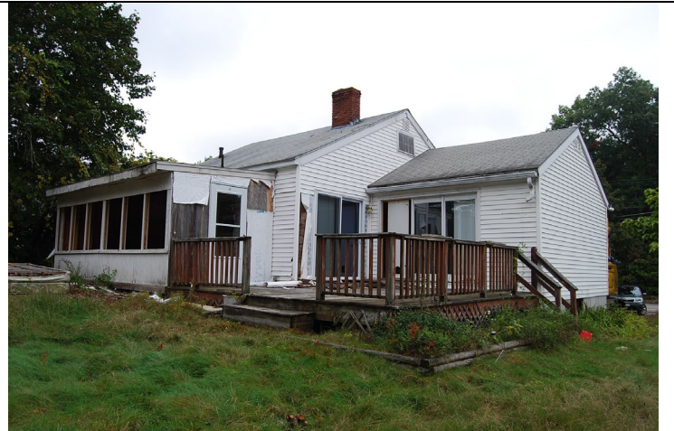
View looking northwest toward rear (south) and side (east) elevations.
