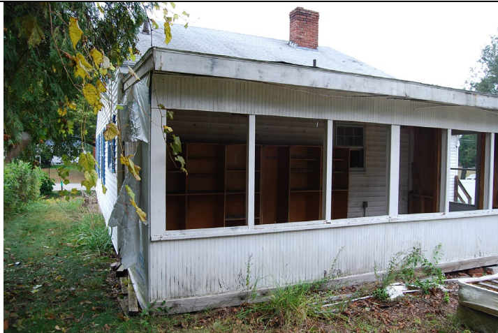
View looking north along west (side) elevation and enclosed porch attached to south elevation.
