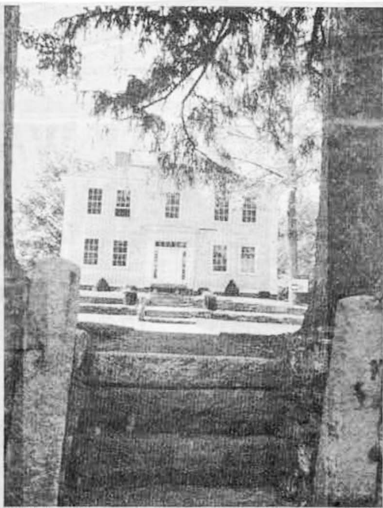
CMFD-BEGINNING A NEW LIFE is the imposing Rev. Hezekiah Packard House on Westford Street, now being completely renovated for private residential use. During its long history it served as a home, a school, and, in part, a plant conservatory which was a novelty at the time. Mr. Packard was a minister, teacher and book-lover who established the Social Library, forerunner of the Chelmsford Public Library which became the Adams Library. After its last use as a multi-family dwelling, it stood vacant for many years but was in the process of restoration when sold several months ago. (Photo by Jean Sougnez)
