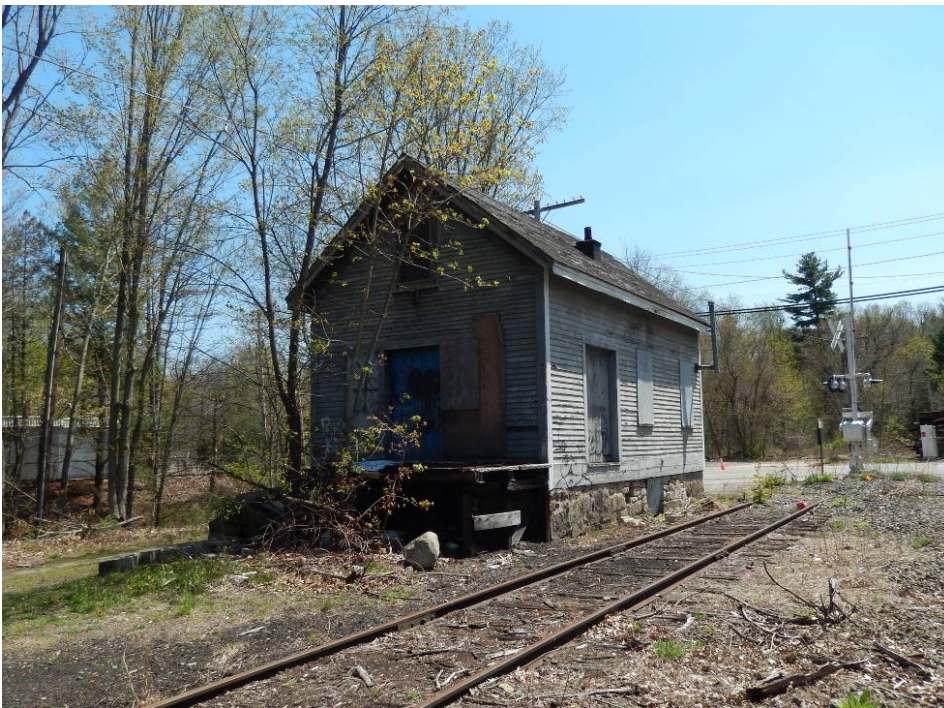
Rear of freight house, facing south. May 2016.
