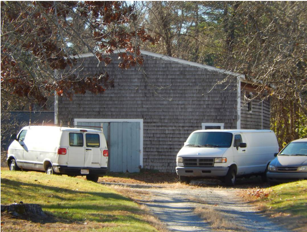
Garage, facing west. November 2015.
