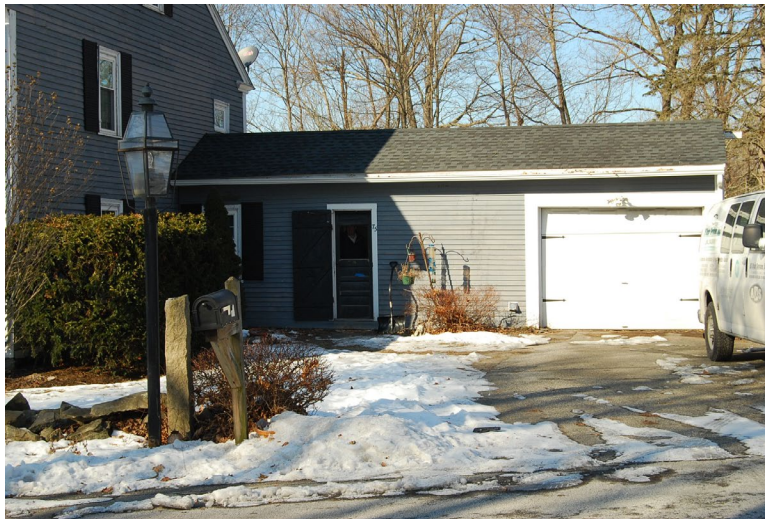
East ell. View looking north.
