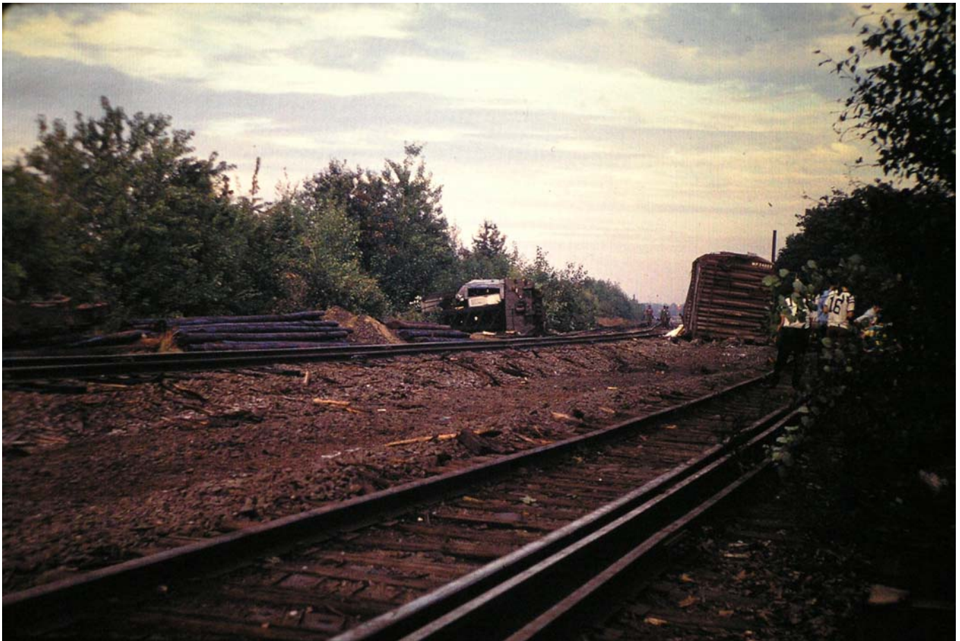
Wrecker crane not properly stabilized rolled over and killed operator
