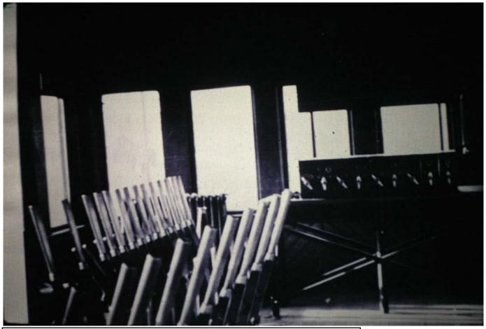
Switch control levers in the control tower - courtesy of John A Goodwin
