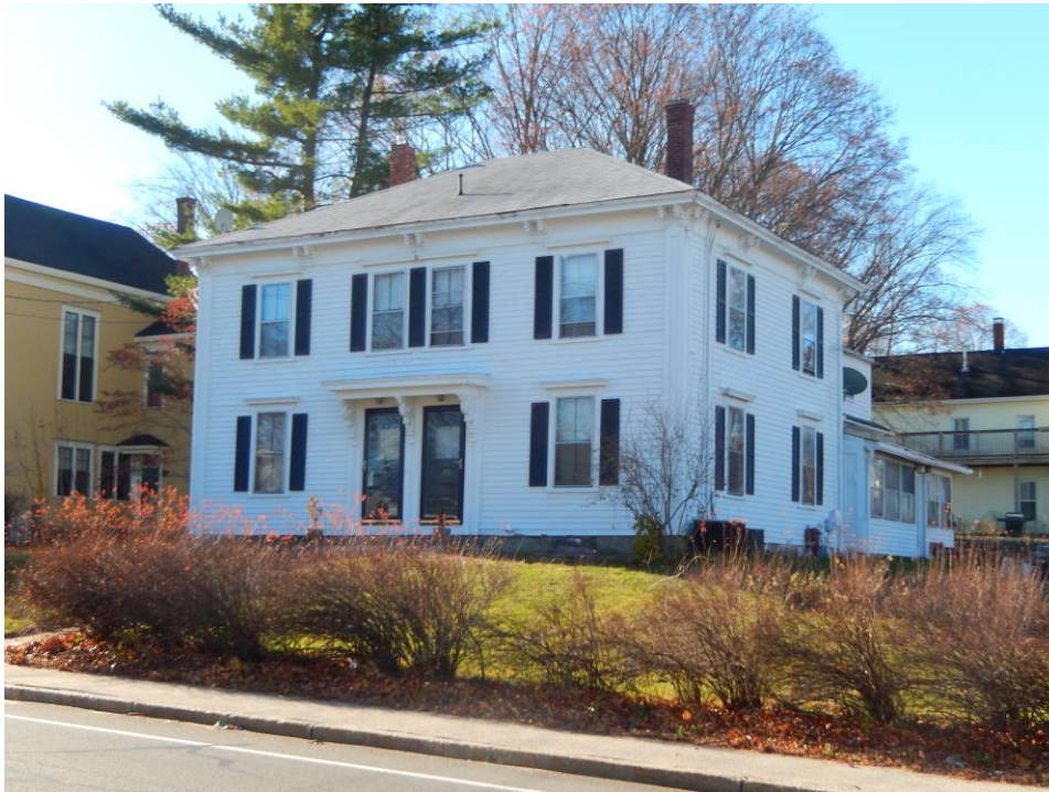
25-27 Princeton Street, facing south. November 2015.
