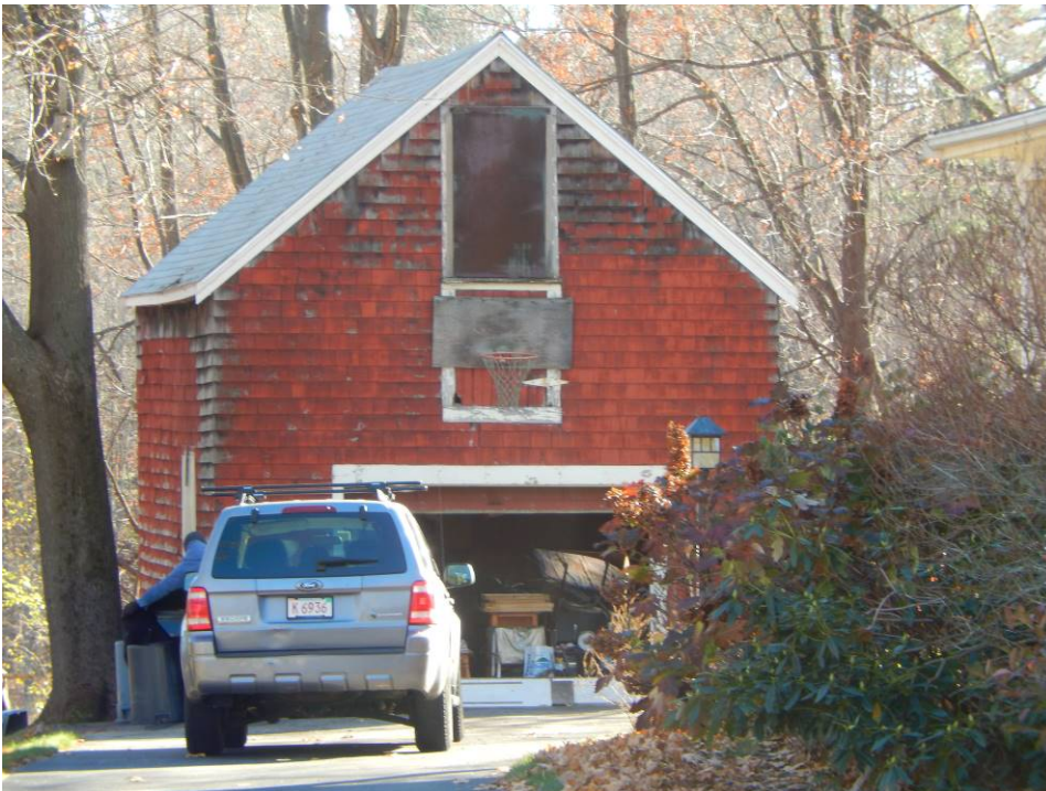
Garage, facing southeast. November 2015.
