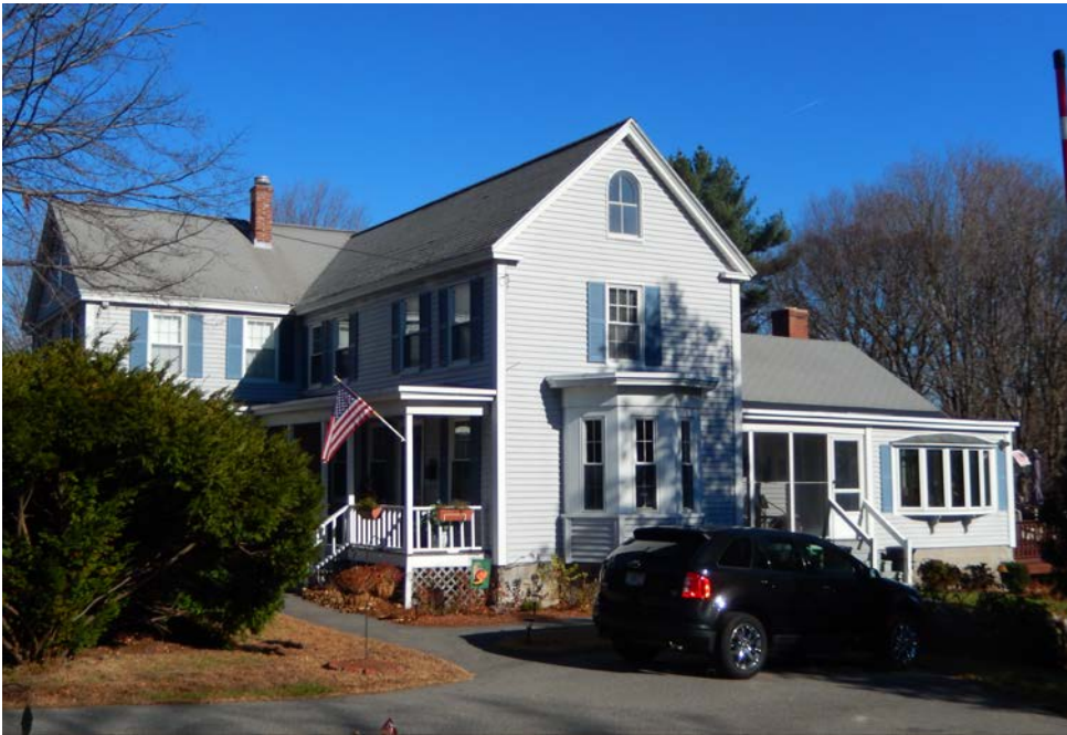
Side view of 186 Main Street, facing northeast. November 2015.
