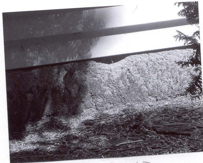
main house foundation Ell foundation is concrete
