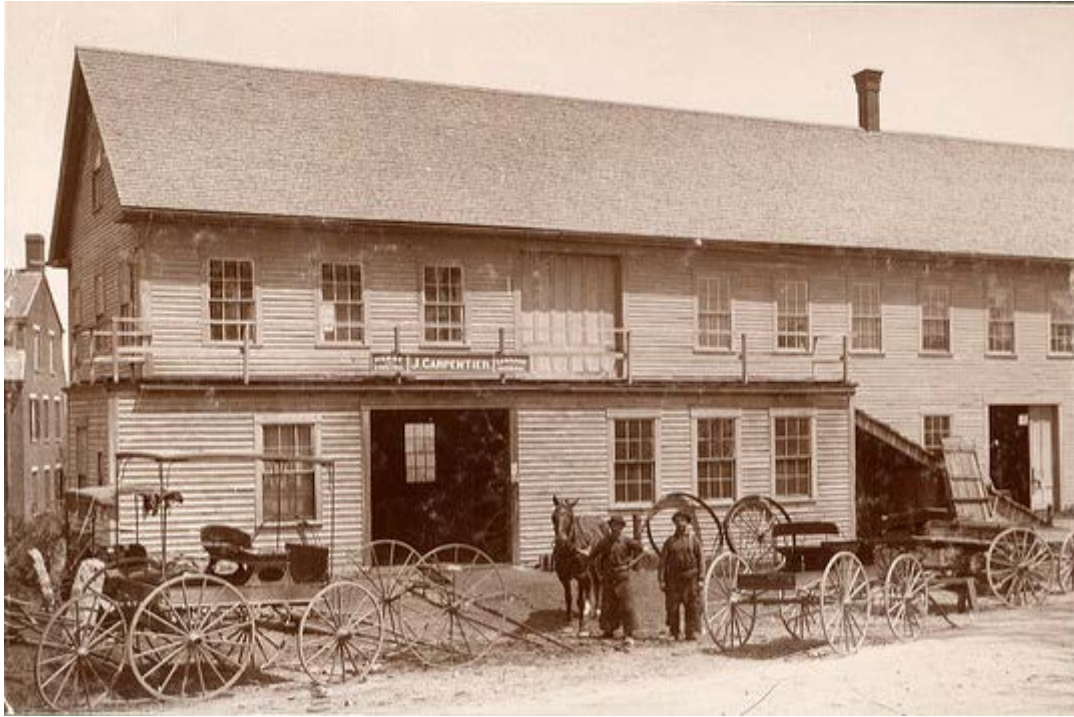
Photograph of the building taken during Joseph Carpentier's period of ownership (1906-1911). (Chelmsford Public Library – Royal Shawcross Photographs Collection.)
