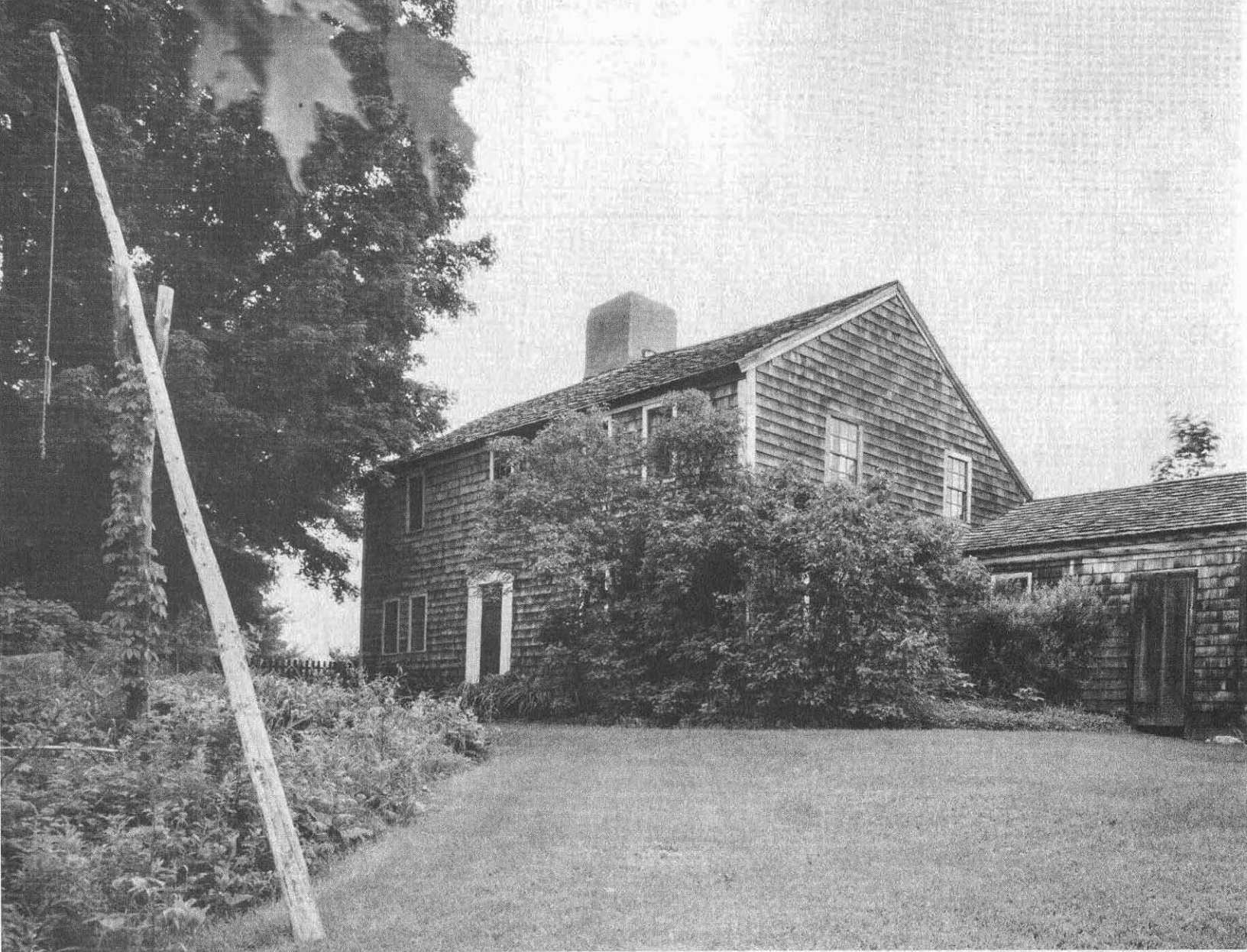
The Well Sweep, Garrison House
