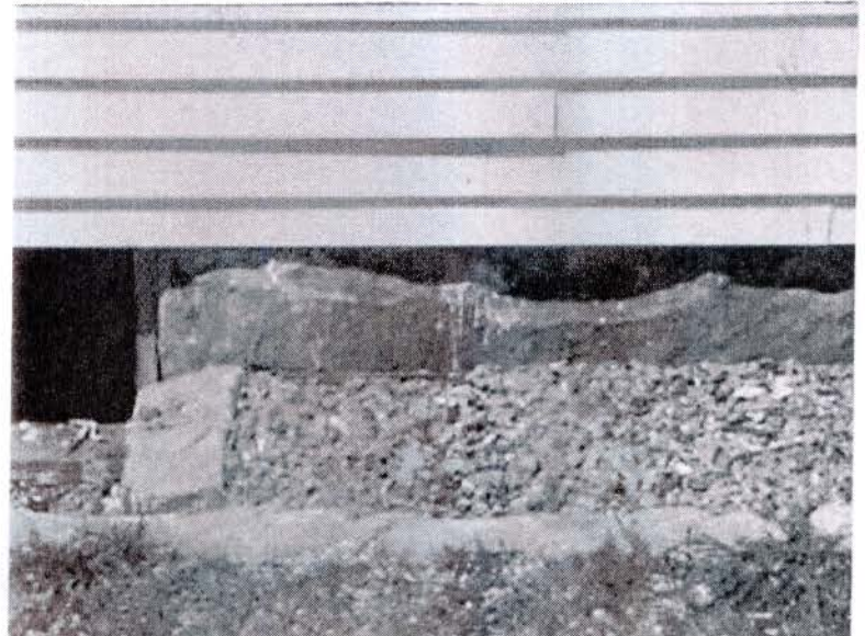
Huge foundation boulders were brought from 155 Boston Rd
