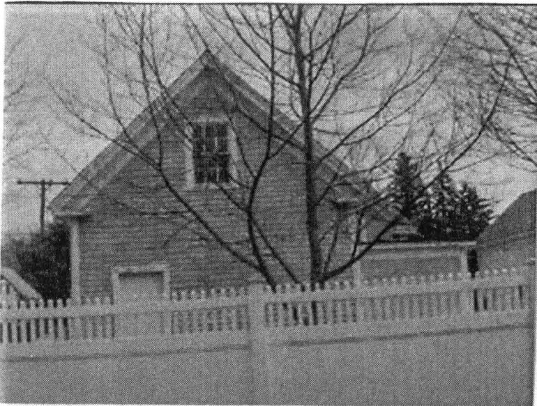
Rear of Barn
