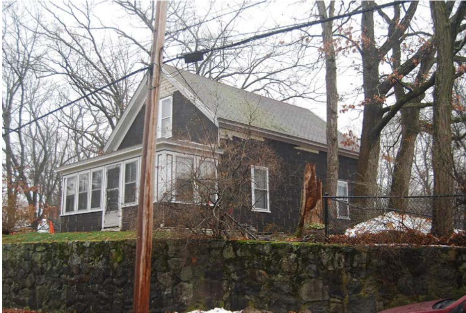
North and west elevations. View looking southeast.
