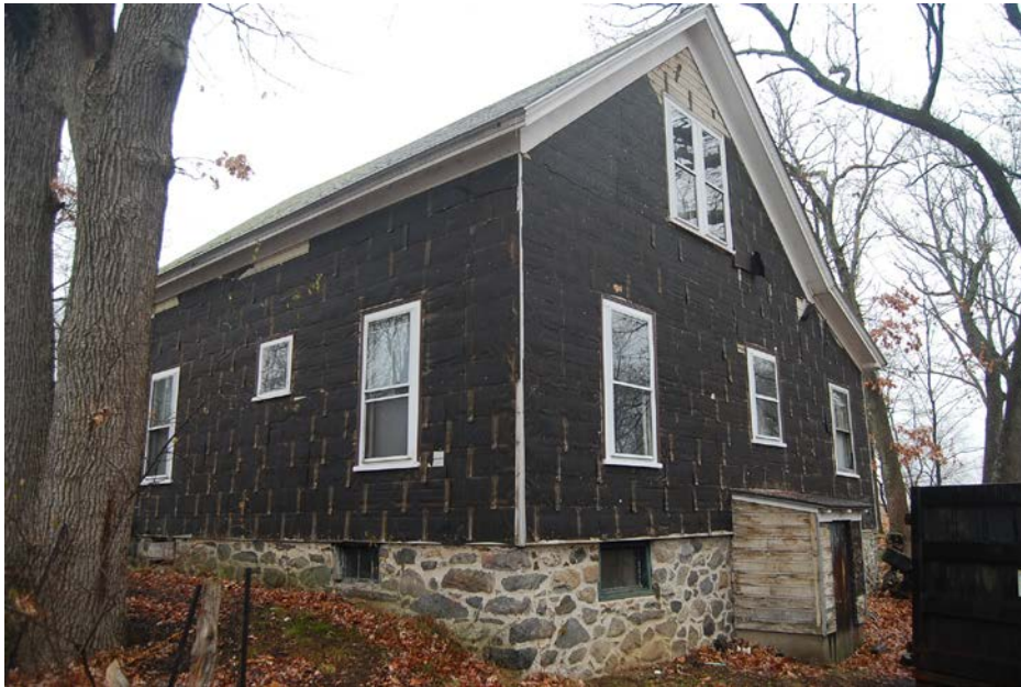
West and south elevations. View looking northeast.
