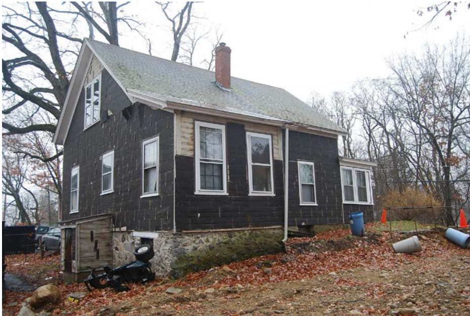
South and east elevations. View looking northwest.
