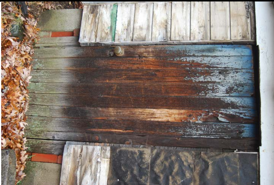
Door to basement level. South elevation.
