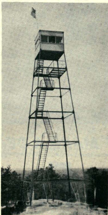
Robins Hill Tower used as a fire lookout for miles around.
