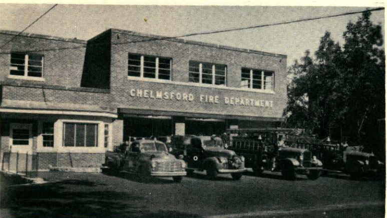
CHELMSFORD CENTER FIRE STATION AT NORTH ROAD.
