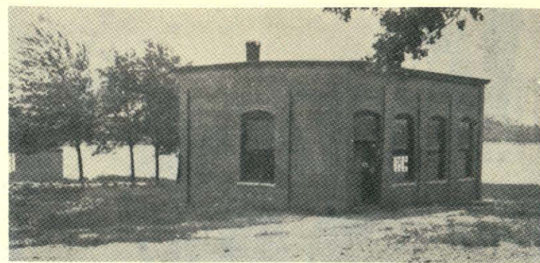
Pumping station operated by the North Chelmsford Water District.
