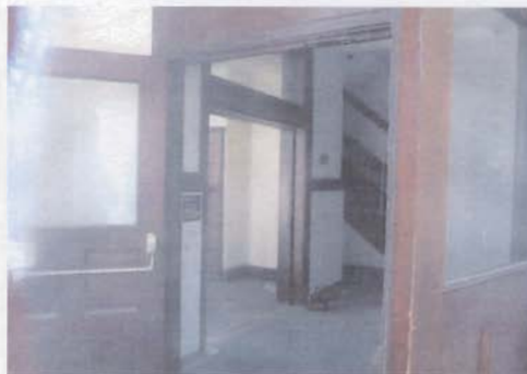
A View of the Inside of MCTS
