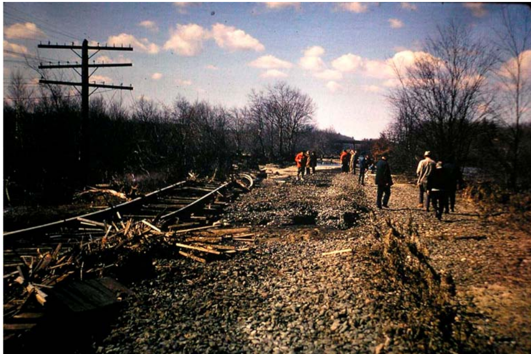
Crystal Lake Dam break April 4, 1970, Stony Brook Railroad track washout and Route 3 overpass (Photo by John A. Goodwin)
