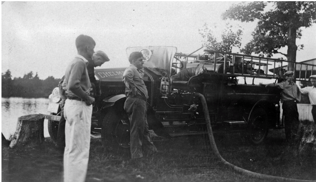
The 1926 Maxim 500 g.p.m. Pumper Engine No. 1, shown here pumping water from a lake It became Engine 4 at East Chelmsford when the 1935 Maxim 500 arrived at the Centre The people were not identified (Chelmsford Fire Department Collection)
