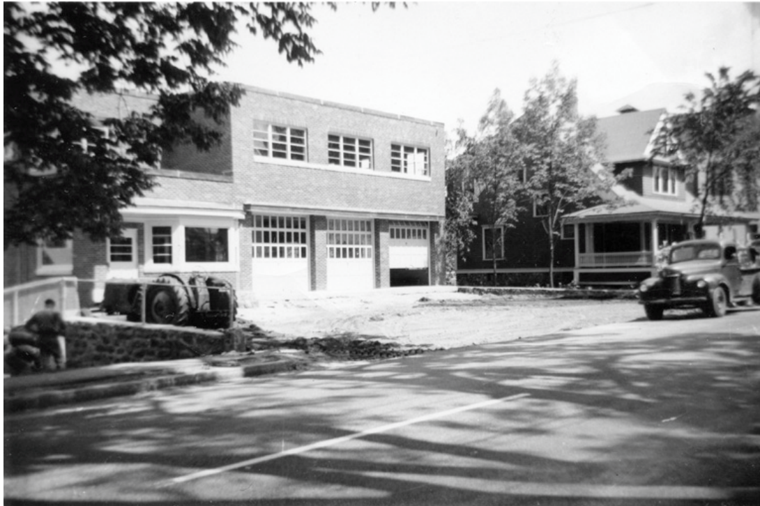
1953 Grading the apron in front of Center Fire Station (Chelmsford Fire Department Collection)
