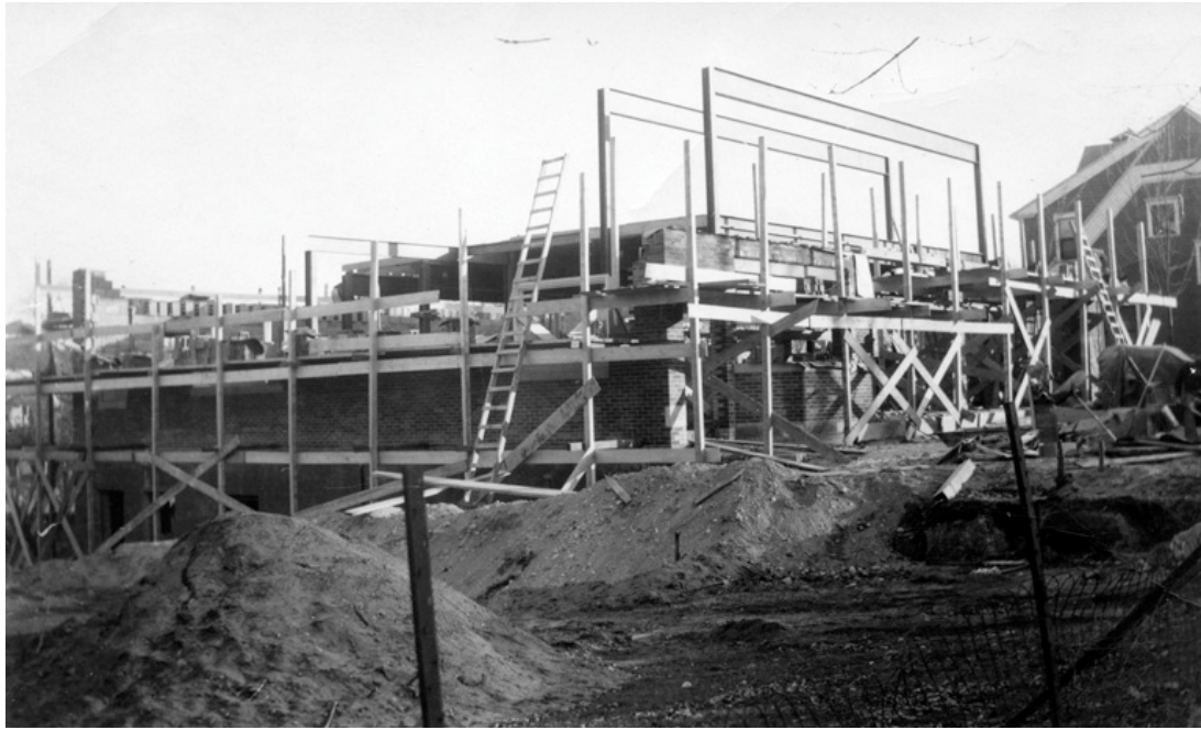
1952 Masons building the first floor of the Center Fire Station (Chelmsford Fire Department Collection)
