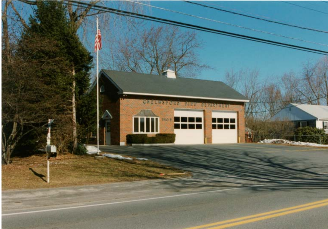
The South Chelmsford Fire Station was opened in January 1967 (1995 photo, Chelmsford Fire Department Collection)
