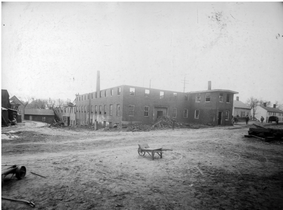
1901 Silver & Gay Machine Shop Fire from across Foundry Street (Chelmsford Public Library Collection)
