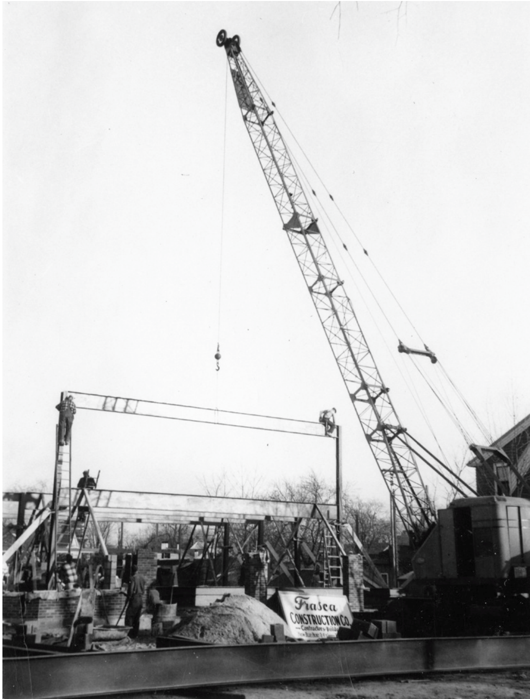
1952 Installing steel for the the Center Fire Station engine bays and second floor (Chelmsford Fire Department Collection)
