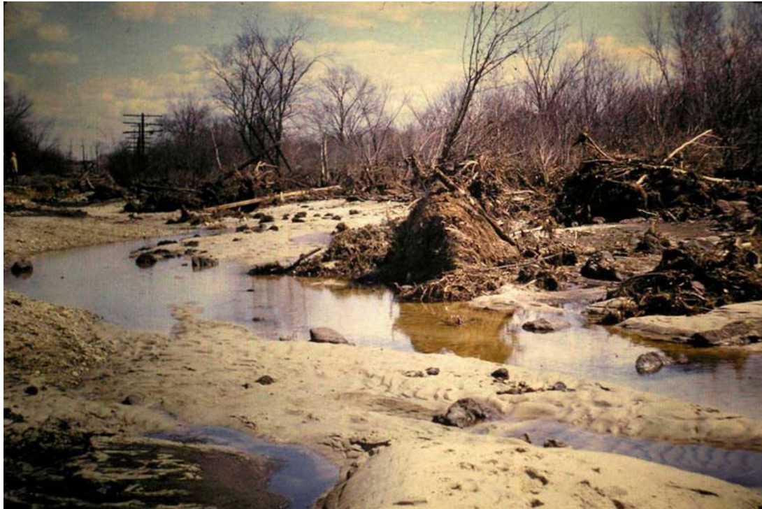
Crystal Lake Dam break April 4, 1970, destruction of the Stony Brook Railroad bed below the dam (Photo by John A. Goodwin)
