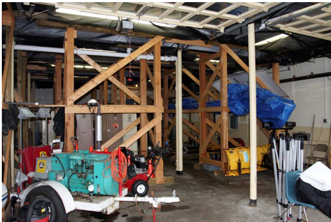
Center Fire Station floor bracing under the engine bays (Photo by Fred Merriam)
