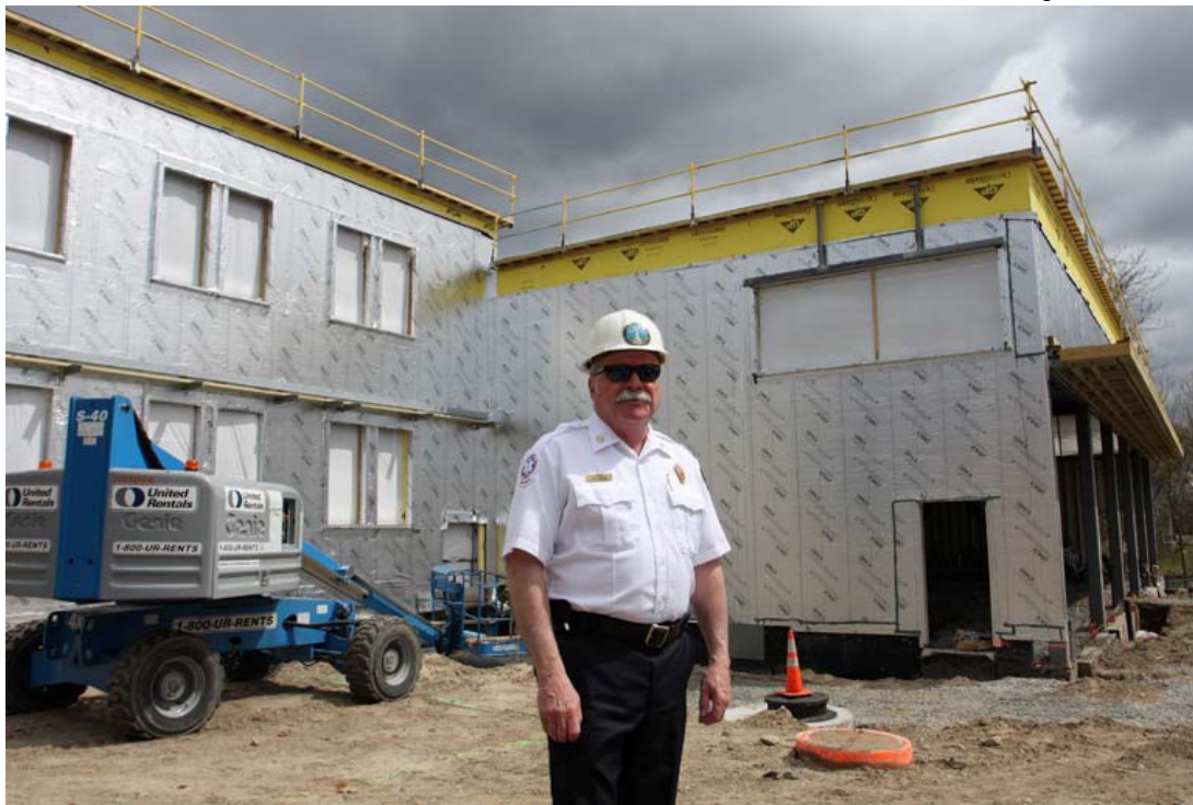
Chief Curran visiting the fire station construction site at 50 Billerica Road on May 5, 2014 (photo by Fred Merriam)
