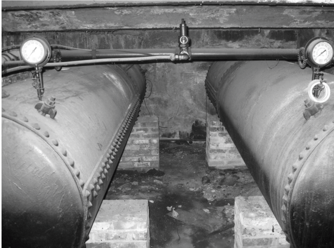
The 1923 air tanks for the Town Hall fire whistle (2009 photo by Fred Merriam)
