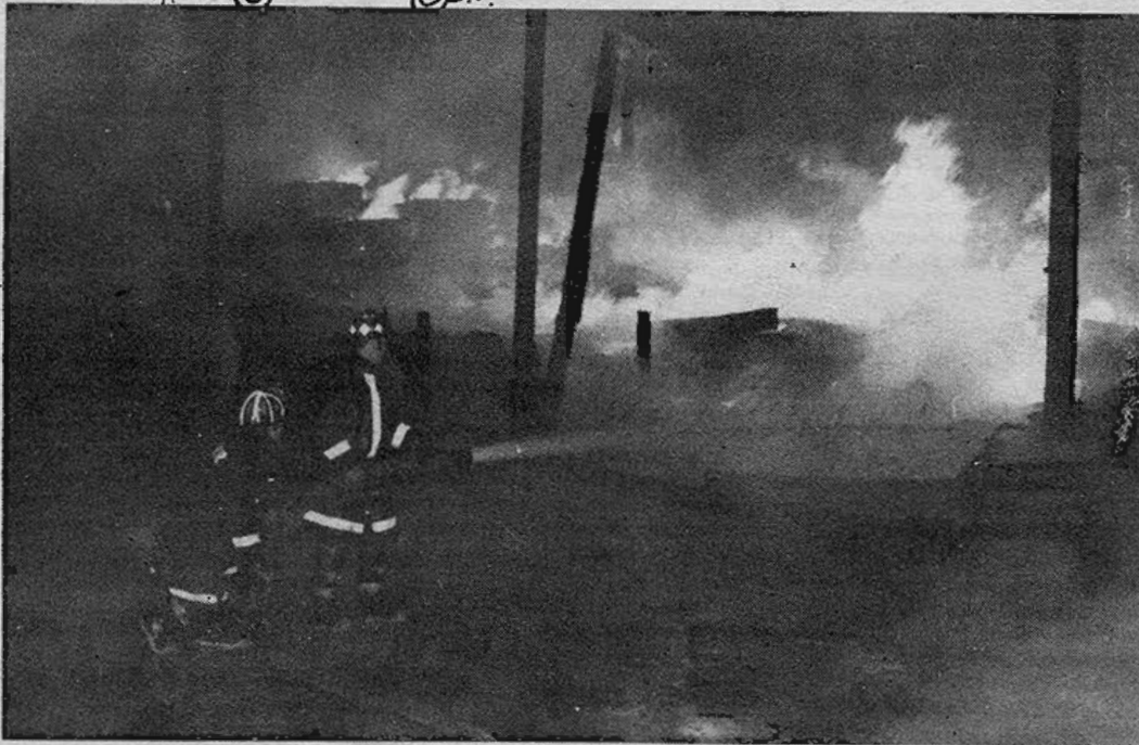
CMFD-THE OFFICE AND THE LARGE STORAGE SHED, filled with bundles of shingles and lumber of many kinds, burned for hours after the fire was discovered on Friday night, Dec. 22, at the State Line Lumber Co., Cushing Place, Central Square. Here firefighters are working near the storage section of the 160 foot building, piled high with building materials. (Photo by Tec Art Photography)
