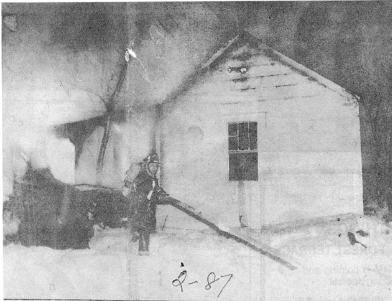
Alarm Fire —Chelmsford firefighters spray water onto the rear of a home (left) at 91 Locke Road early last Thursday morning. In photo at smoke creates an eerie haze around the
