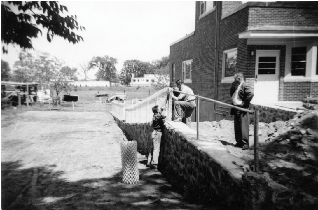
1953 Installing the chain link fence beside the Center Fire Station (Chelmsford Fire Department Collection)
