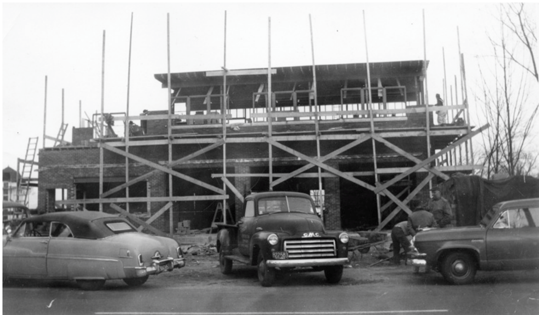
1952 Masons building the second floor of the Center Fire Station (Chelmsford Fire Department Collection)
