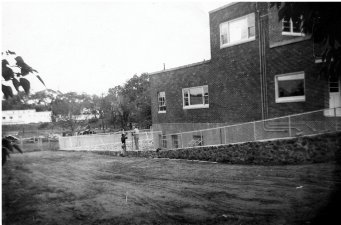
1953 Finishing the chain link fence beside the Center Fire Station (Chelmsford Fire Department Collection)
