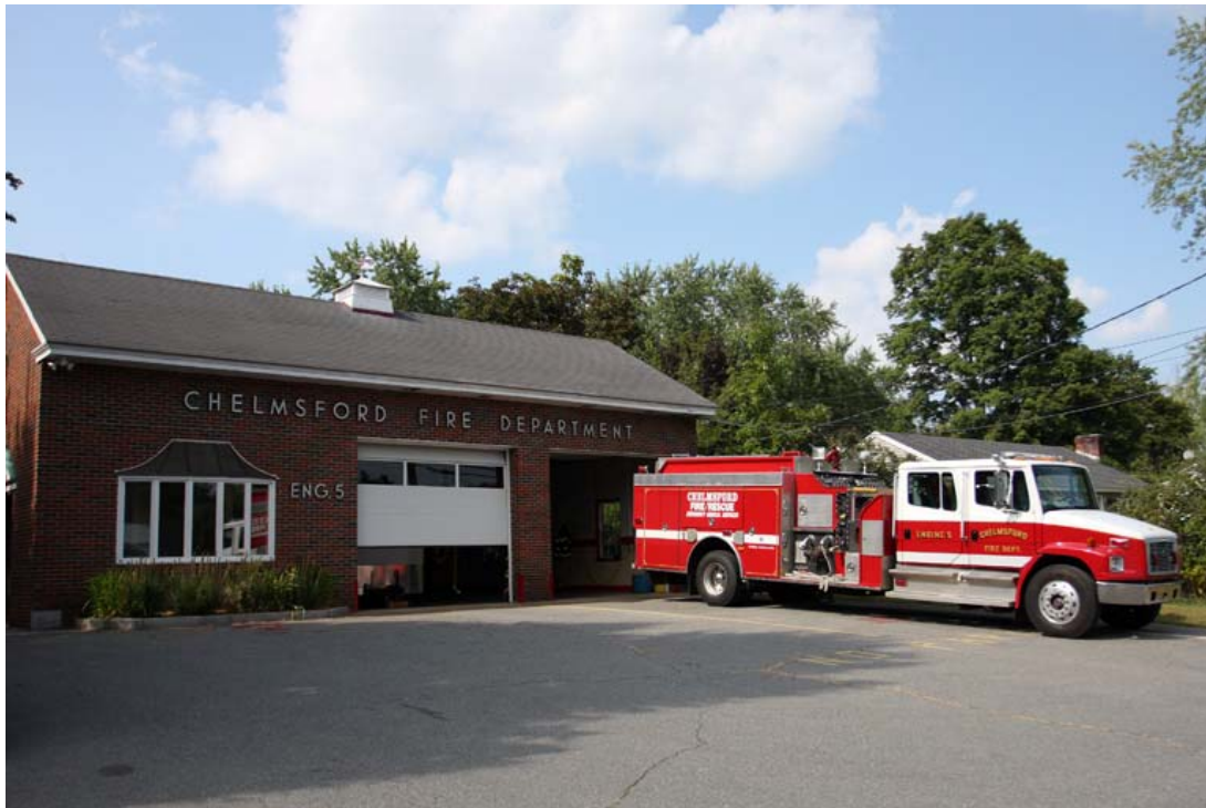
South Chelmsford Fire Station re-opened in October 2011 (2013 photo by Fred Merriam)
