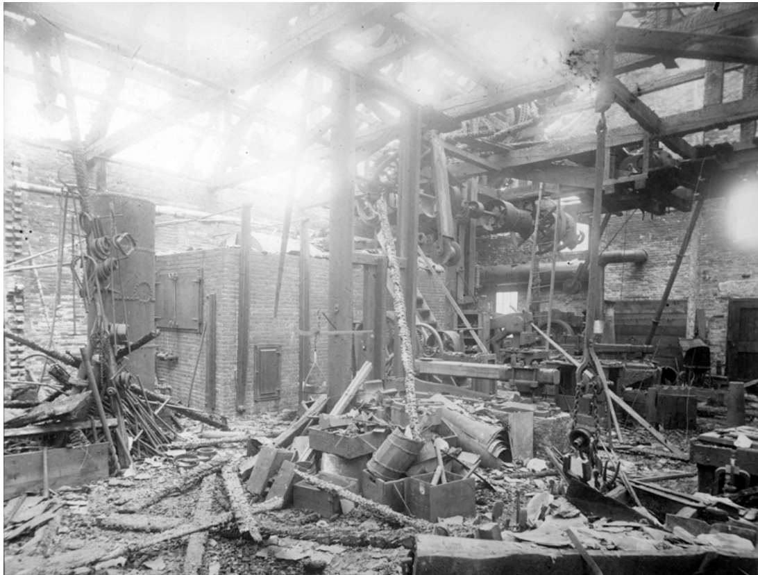
1901 Silver & Gay Machine Shop Fire interior damage (Chelmsford Public Library Collection)
