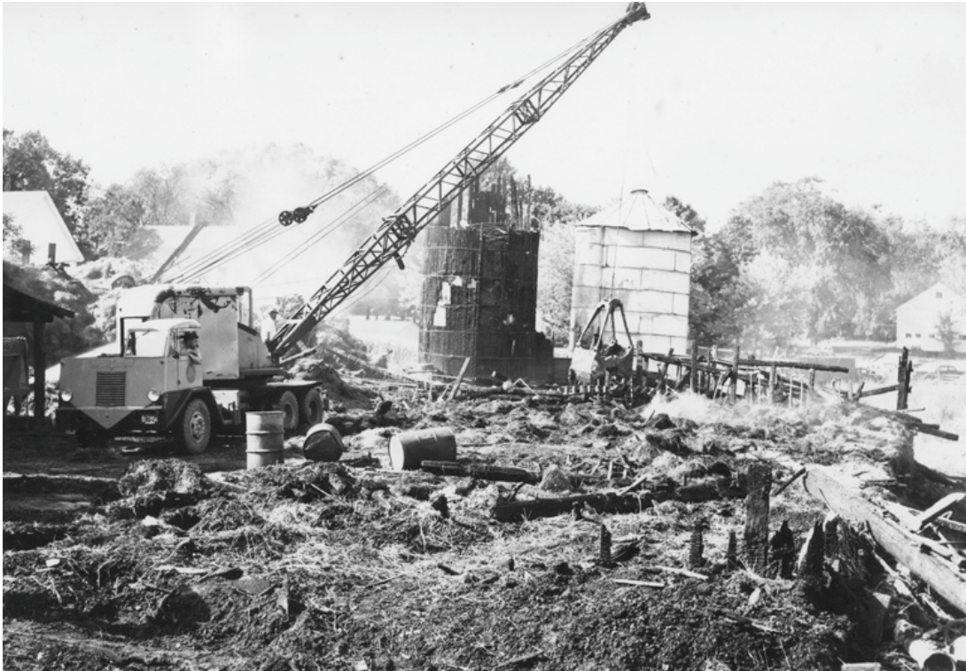
September 1951 Emerson rubble cleanup behind 11 North Road (Chelmsford Fire Department Collection)
