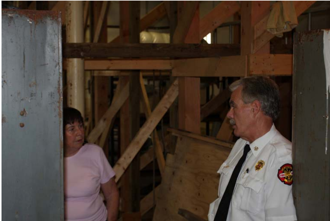
Chief Parow talks with Peggy Dunn about the temporary Center Fire Station repairs at August 12, 2009 open house (photo by Fred Merriam)
