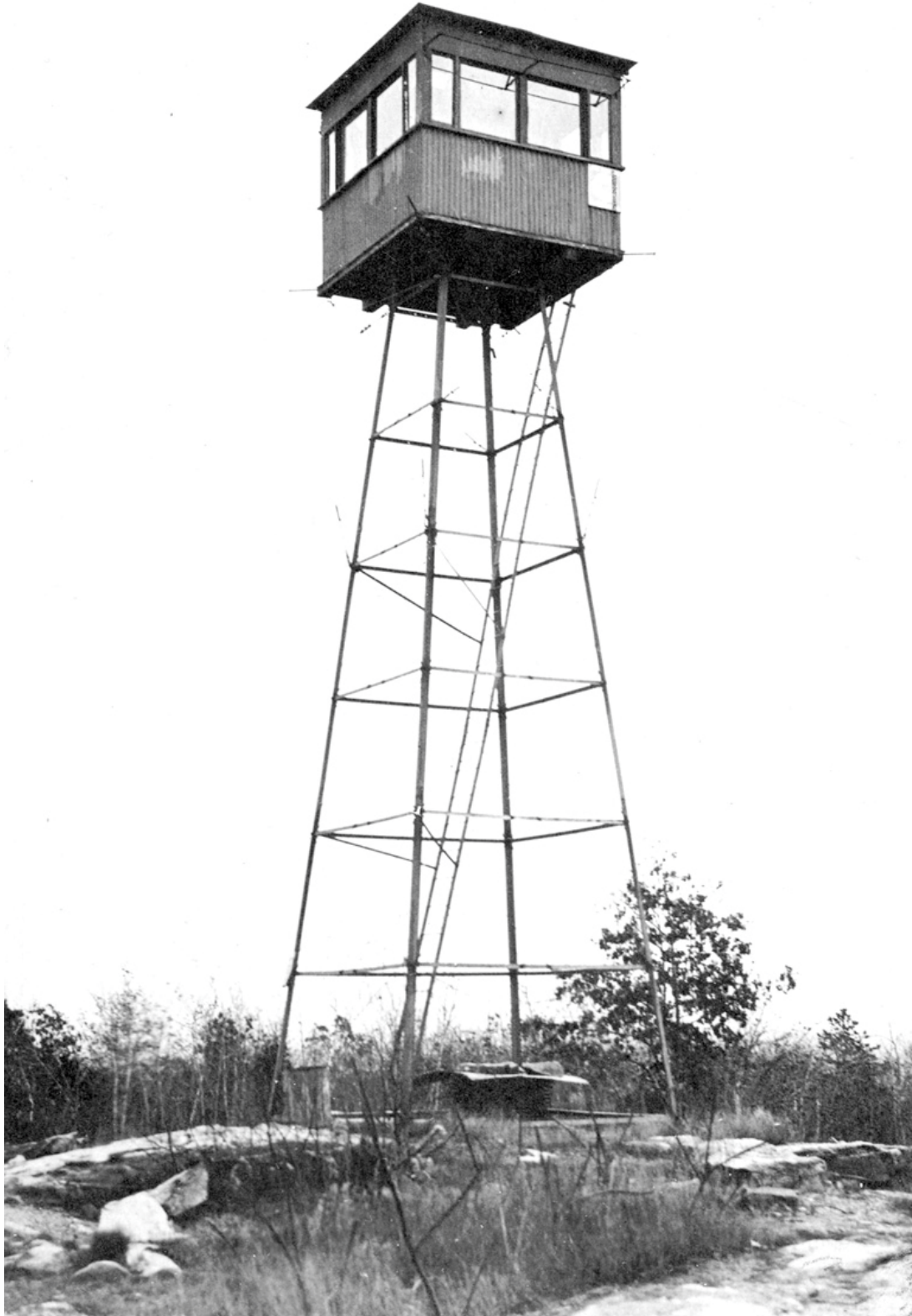
The experimental State Fire Tower on Robins Hill 1911-1918 (Chelmsford Historical Society Collection)
