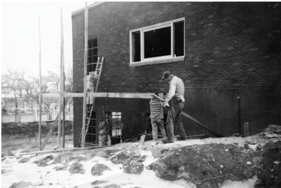
1953 Finishing the side of the Center Fire Station before grading (Chelmsford Fire Department Collection)
