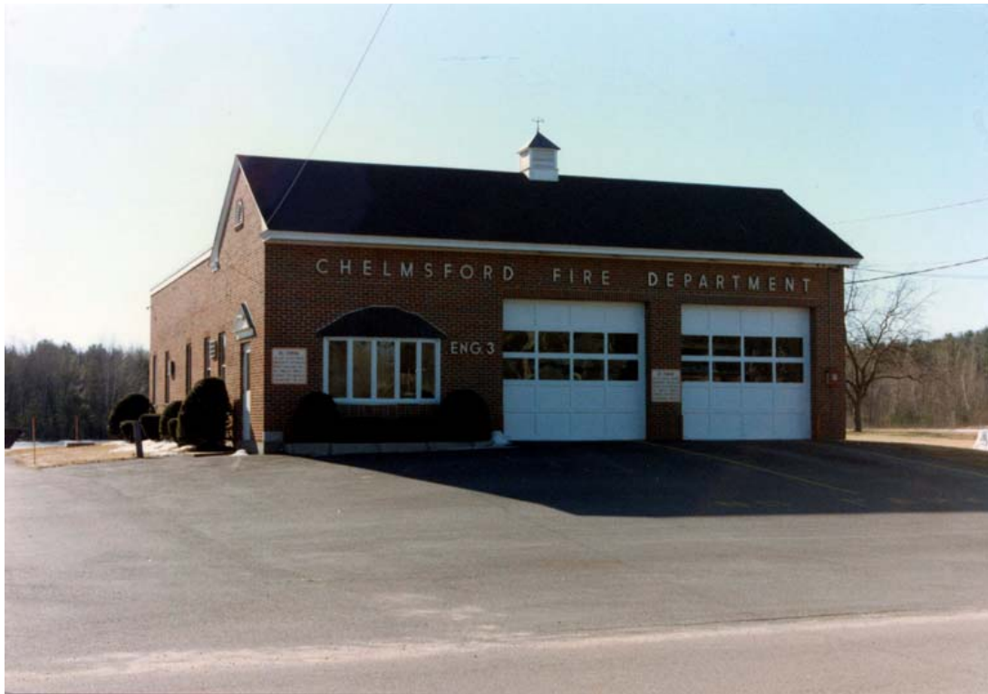
West Chelmsford Fire Station in February 1995 (Chelmsford Fire Department Collection)
